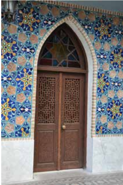
Fig. 6: The facade of the historical bathhouse with a glazed mosaic
