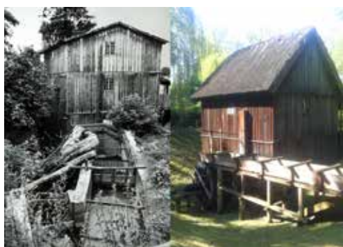
Figure 4: Watermill from Strzygi with: a turbine (left – in situ in 1960s) and a overshot waterwheel (right – ex situ in 2014). Currently in the Ethnographic Museum in Toruń (photograph by Archive MET, sign. I-1306-90; K. Kopczyński 2014).
