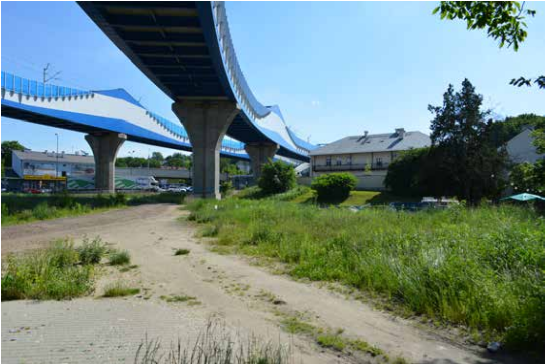
Fig. 2: Museum of Podgórze seen from the perspective of the land under the railway flyover – future park. Photo: K. Jagodzińska.
