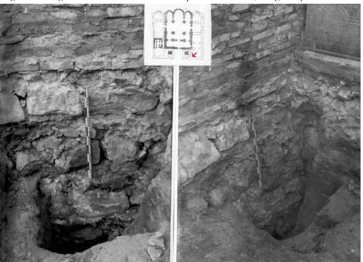
Fig. 4: The Dormition Cathedral. Excavation site no. 20 b. Pit in the north-western corner of the southern vestibule to determine the footing level. Photo: [in:] Collection of the Ukrrestavratsiia Corporation.
