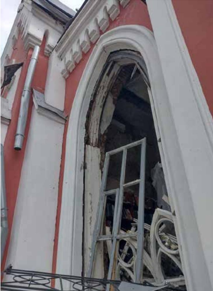
**Figure 5:** *Destroyed window of the courtyard facade.* Photo by A. Glushchenko, 2022
