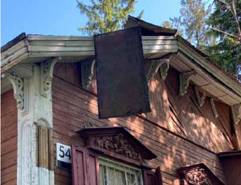
**Figure 7:** *Damage to the corner fragment of the facade of the “wooden Art Nouveau” style mansion. Photo by A. Hlushchenko*
