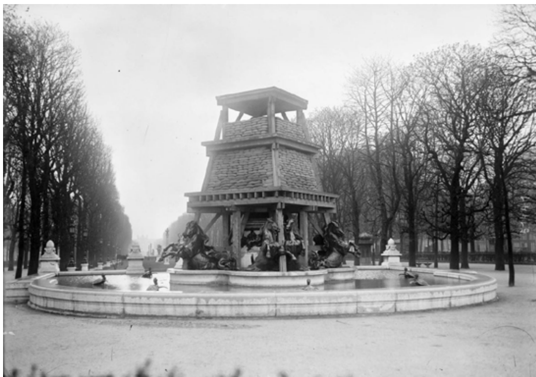
Figure 2: Structure with bags to protect the Quatre-Parties-du-Monde fountain in the Jardin Marco Polo in Paris from German bombing, 1918.
